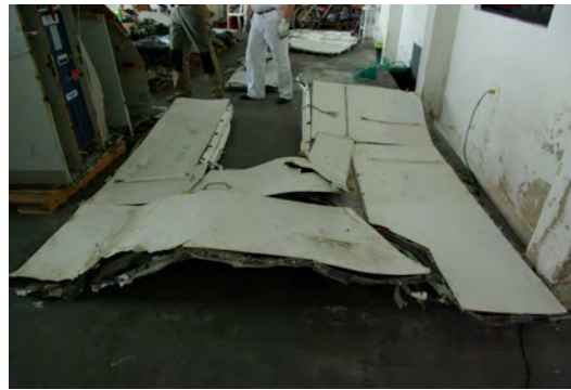
Figure 39: Ceiling of the LDMCR: with top-downwards deformation
